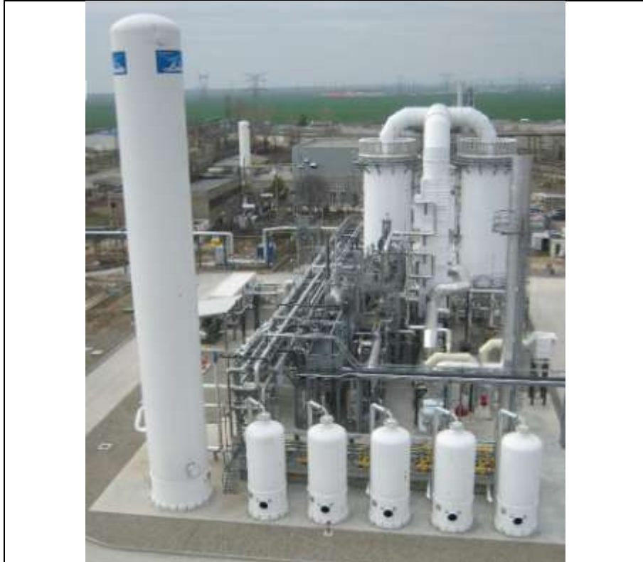
2 reformere; 5 adsorbere; rezervor azot
